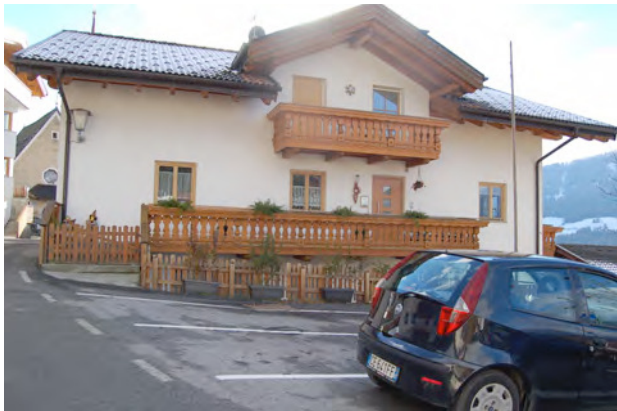
BP Ped 62/2 Westansicht – Vista da Ovest
